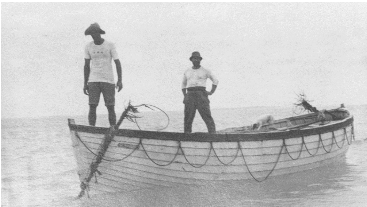
The two severed ends of the “dummy” cable after the attack. Image courtesy of Porthcurno Telegraph Museum.
