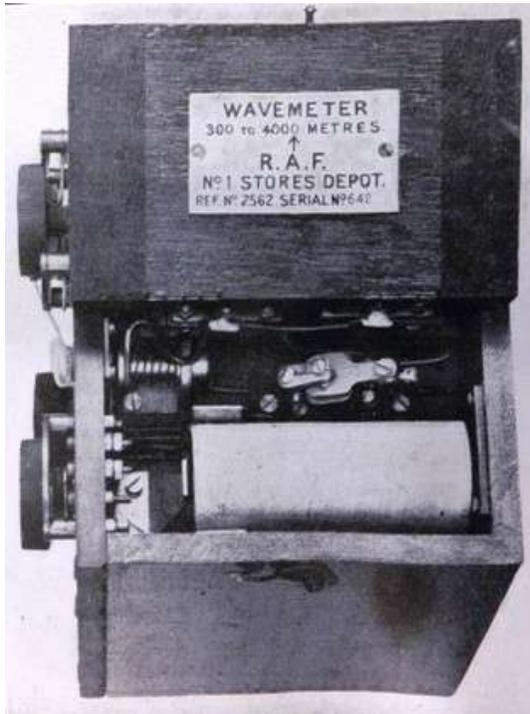
Figure 10. RAF Townsend-type wavemeter.
